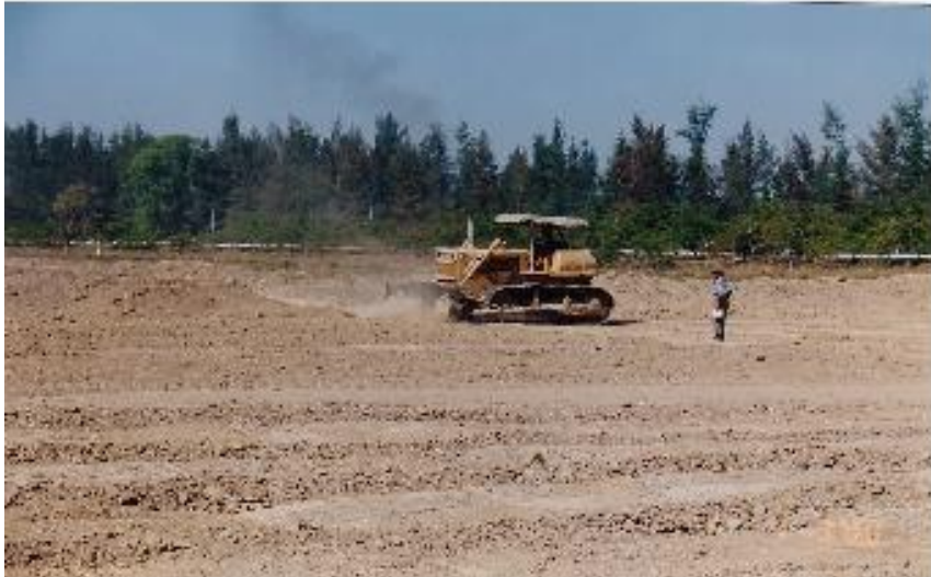
Top Soil Removing
