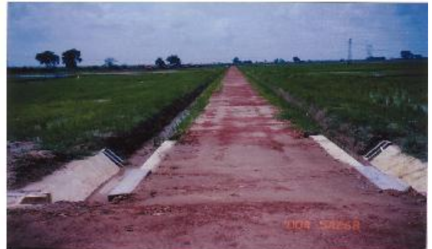
Laterite Branch Farm Road & Water Course
